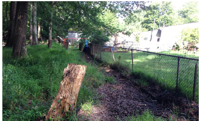
Figure 14. Drainage channel from Petersburg National Battlefield looking downstream approaching S. Whitehill Drive (above) and after taking the 90° turn along the property line (below).
