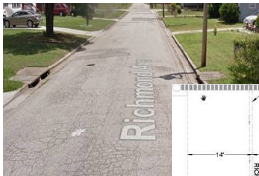
Existing Richmond Road
