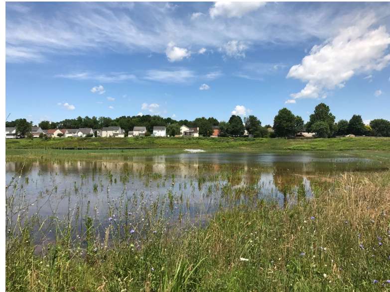
Figure 5. Mulberry Run Constructed Wetland, Waynesboro VA
