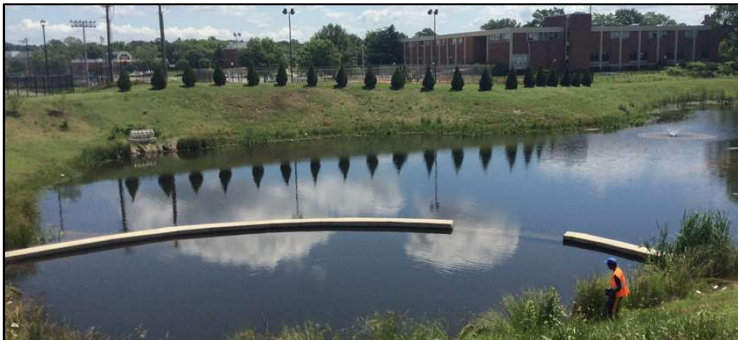
Figure 4. Trojan Stormwater Management Pond, VSU
