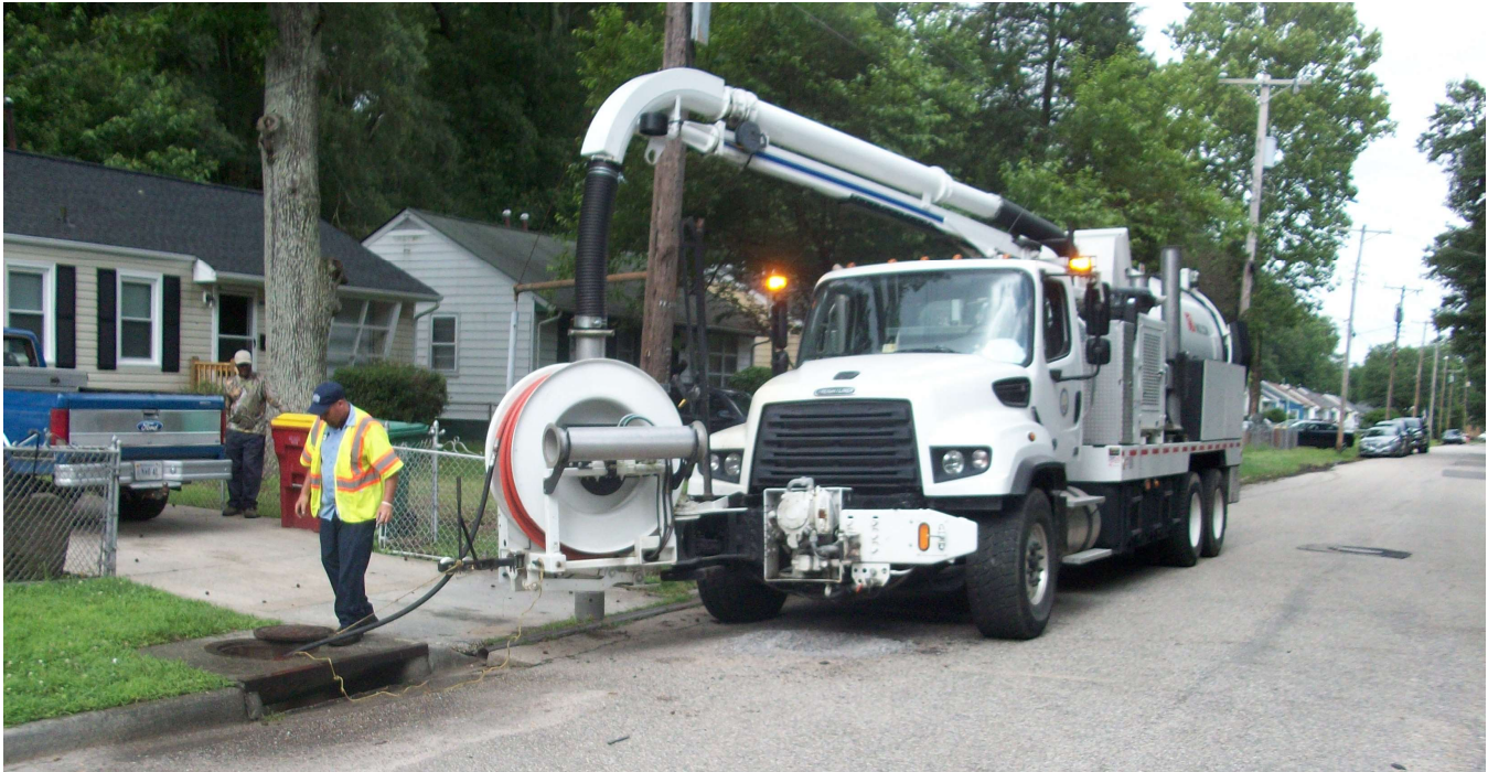
Figure 8. Storm drain cleanout by City Street Operations staff, June 12, 2018.
