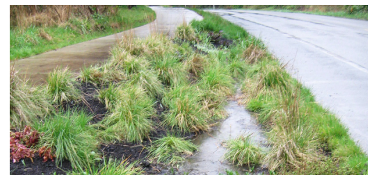
Example of a planted swale during rain event
