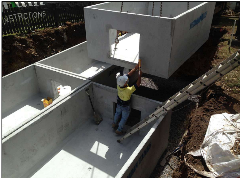
Figure 5. Example Underground Detention Chambers
