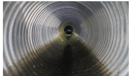
Examples of storm sewer infrastructure installation (top) and an underground detention (above).
