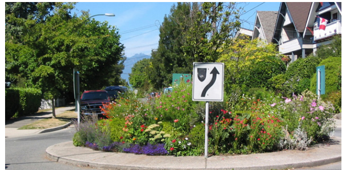
Example of a vegetated traffic circle in a residential neighborhood that slows traffic, collects stormwater and adds aesthetic value. A drainage study will identify whether there is adequate road width and right of way to accommodate a traffic circle.
